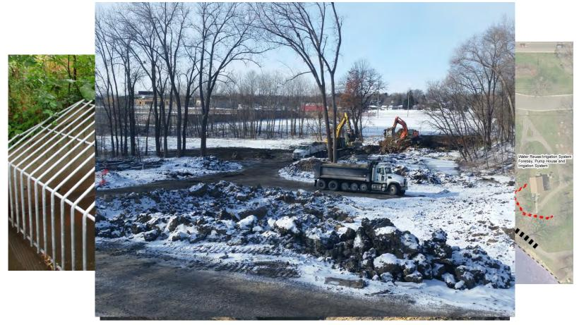
Thompson Lake contaminated sediment removal and stormwater treatment project. 180 acre drainage area will be treated with a stormwater pond, treatment wetland, and water reuse system.
