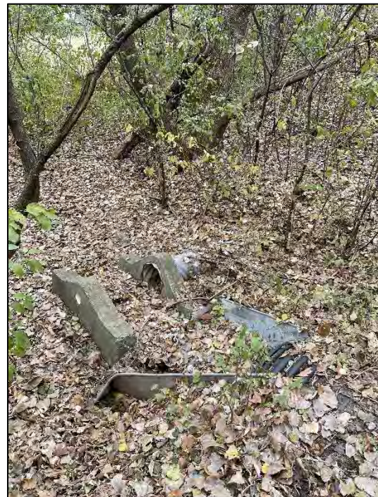
Photo 12 - Outlet from Crown Point BMP
