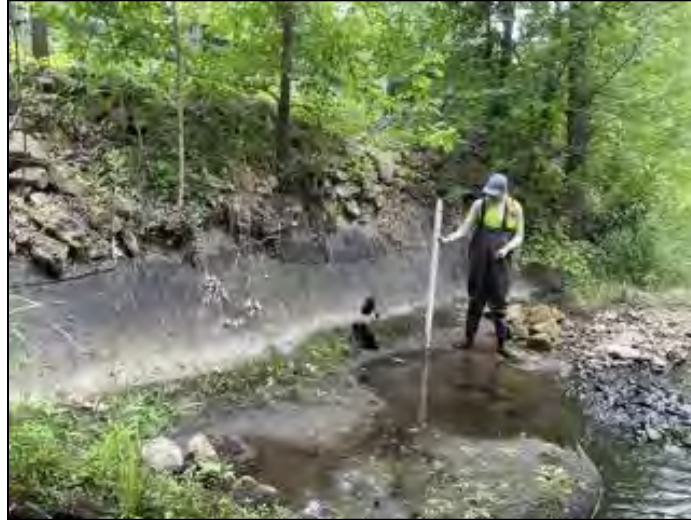
Photo 4: Retaining Wall Below Lilydale Trailhead Parking Lot
