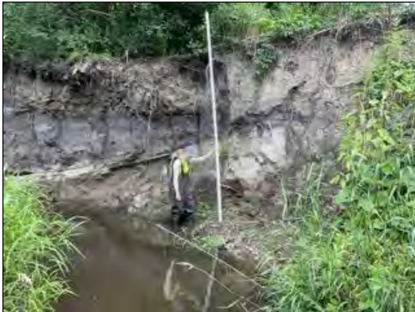
Photo 8: Severe Erosion at Valley Park RTR to Wentworth Site
