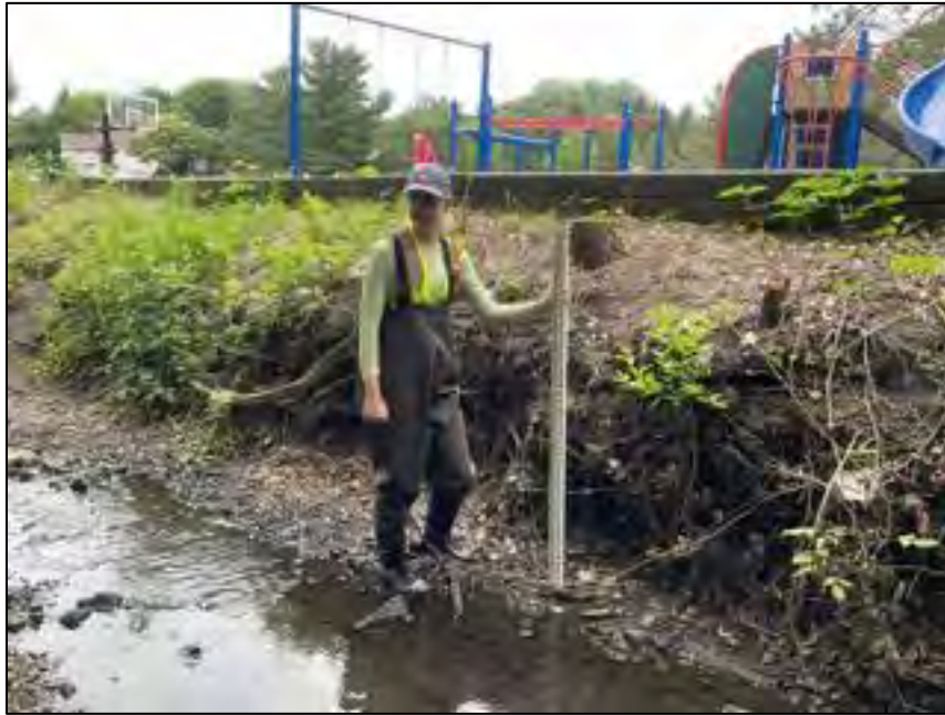
Photo 16: Severe Erosion near Valley Park Playground
