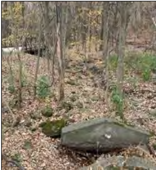
Photo 6: Park Place Storm Sewer Outlet
