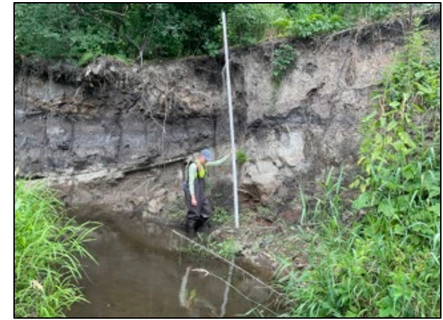
Site 1 – Eroding banks up to 14 feet in height
