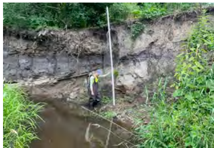
Severe erosion areas along Interstate Valley Creek
