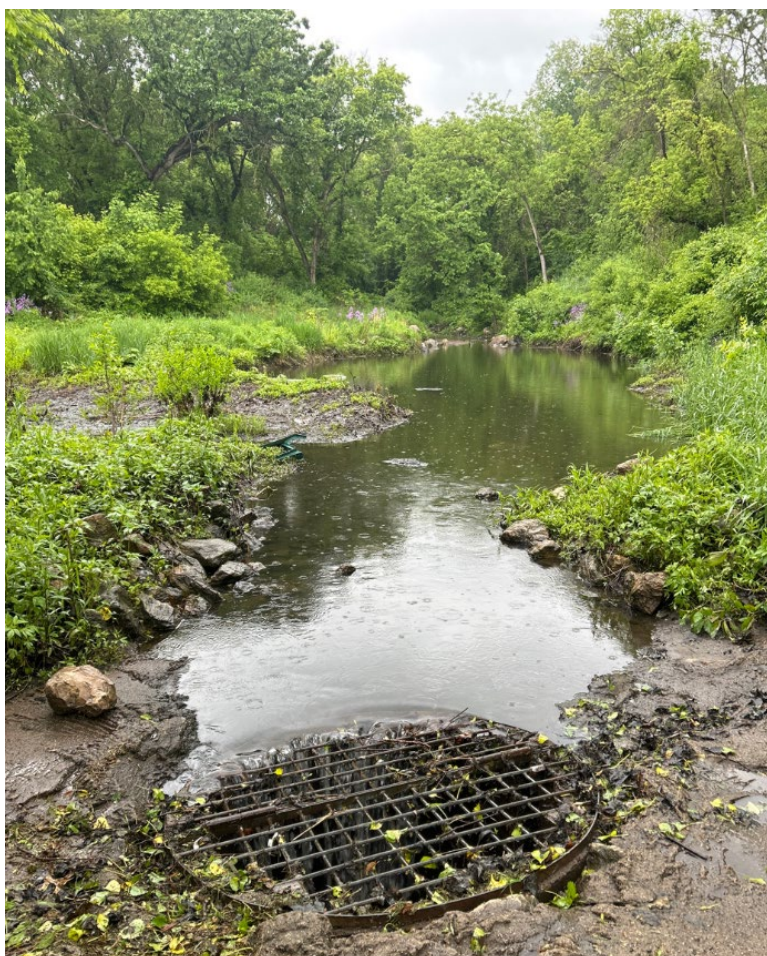
Photo 26 - Existing Gisch Pond outlet structure
