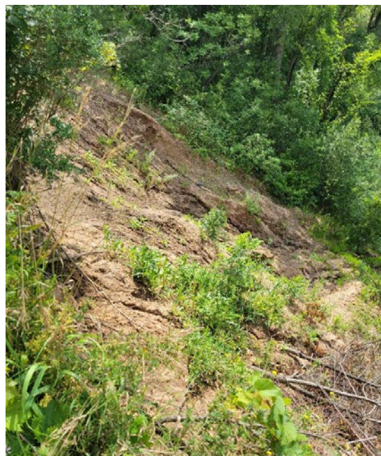
Photo 6- Existing scarp beneath upper Brickyard Trail trailhead
