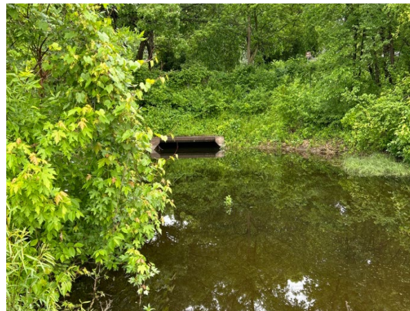
Photo 20 - Existing outfall in River Front Park
