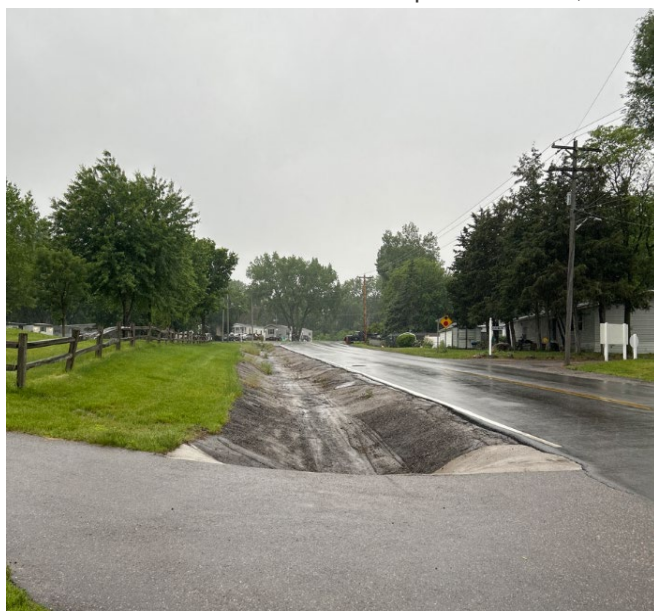
Photo 21 - Paved swale along Ernster Park
