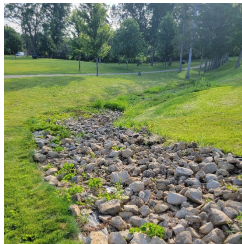
Photo 4 - Existing armored swale in West St. Paul Sports Complex
