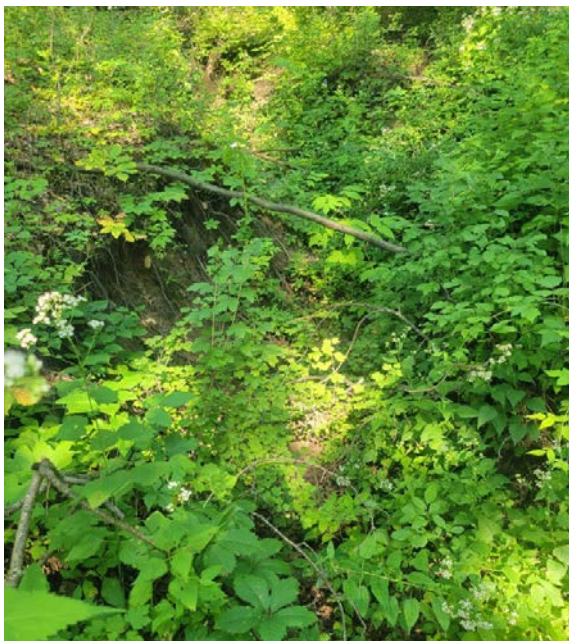
Photo 24 - Vegetated cover over existing ravine downstream of I-State Trucking Pond
