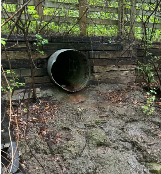
Photo 18 - Outfall with pavement beneath within Dehrer Park Ravine
