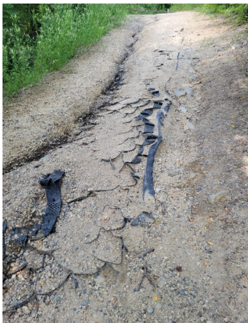
Photo 7 - Geosynthetics in place along Brickyard Trail
